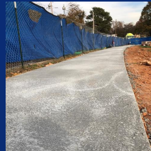
Sidewalk poured along Westhaven
