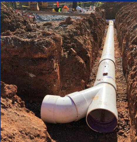
Main level underground MEP - Storm line for roof drains
