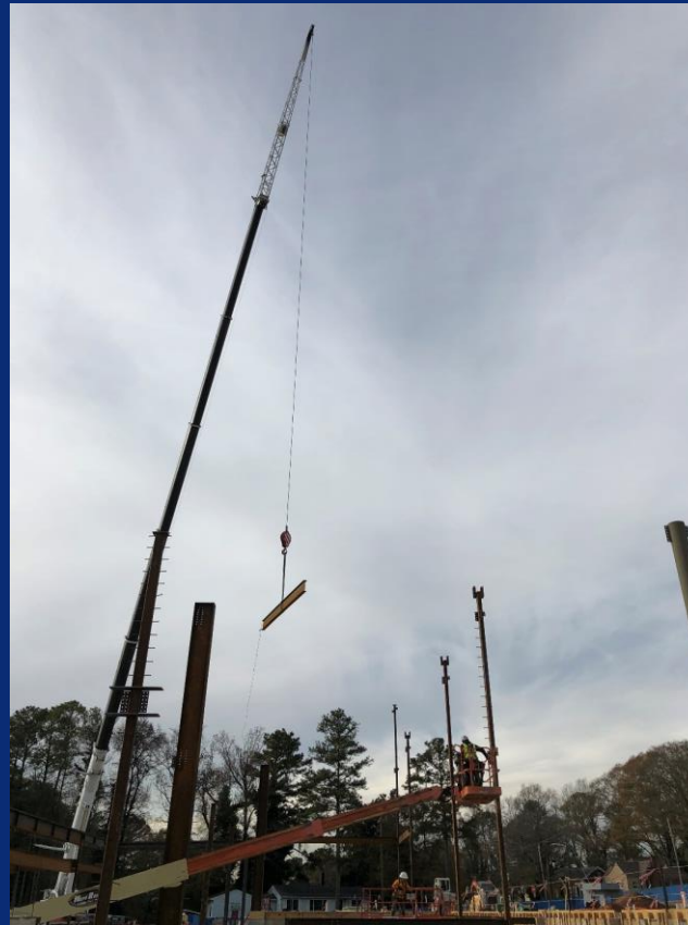
200 ton crane on site flying steel for sequence 1
