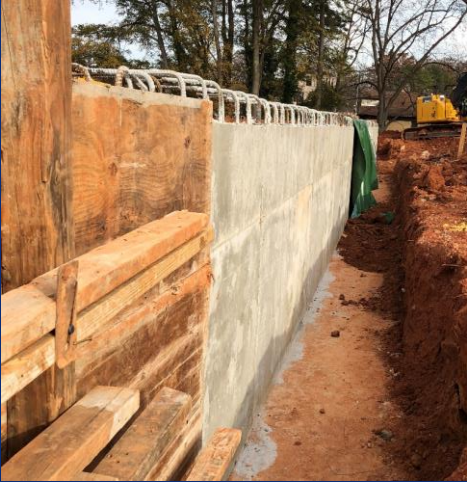
Main level east foundation wall poured
