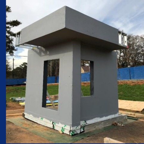
Exterior skin mock-up in progress
